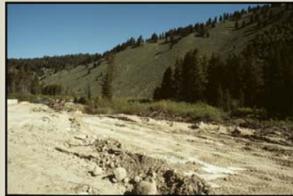
Highway construction in a wetland
