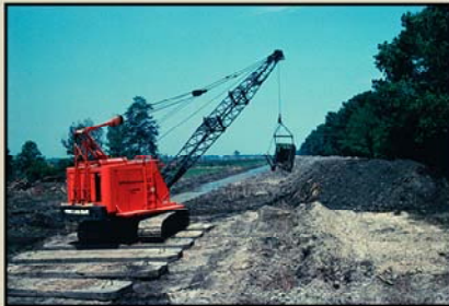
Dredging in a wetland
