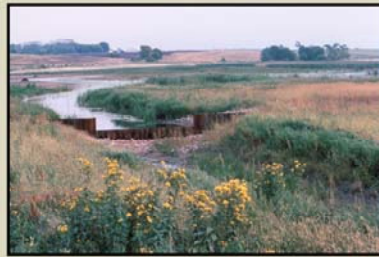
Installation of a water control structure
